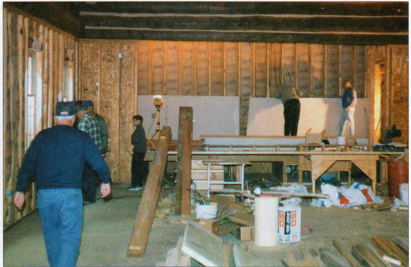
Work continues on new fellowship hall at Williamsport
