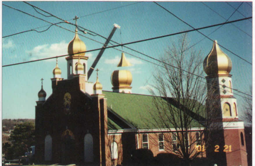
Installation of the newly refurbished cupolas in Pottstown
