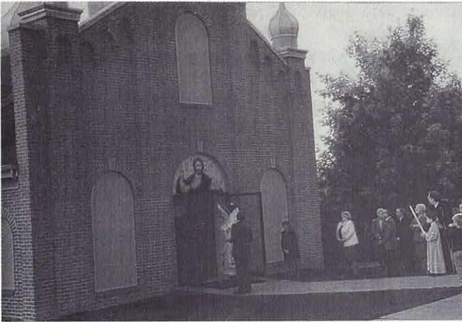
Newly installed mosaic on Holy Trinity Church
