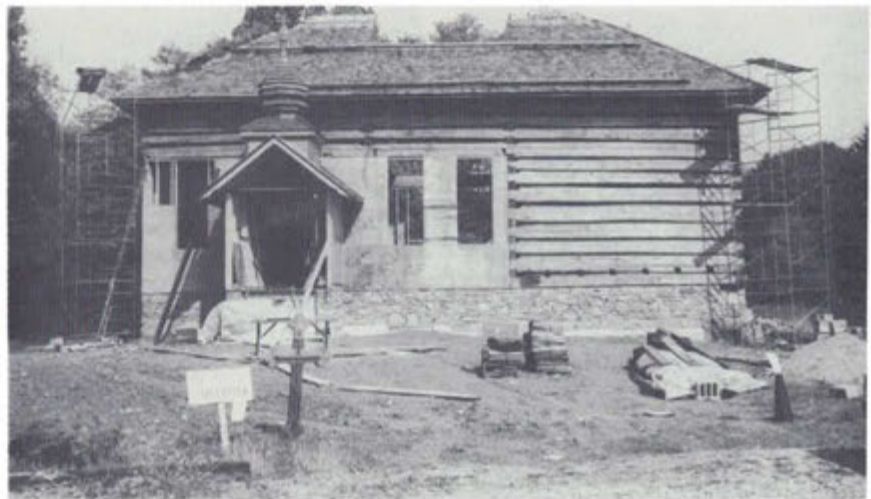
New church under construction for Holy Cross Parish in Williamsport, Pa.
