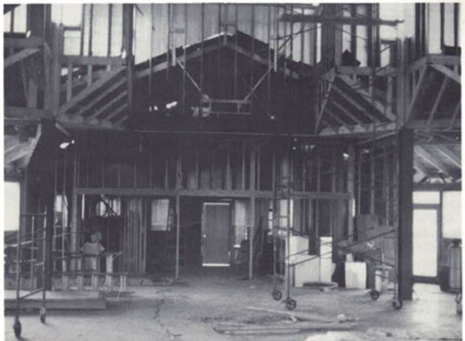
Rear interior view of the new church under construction in Harrisburg.
