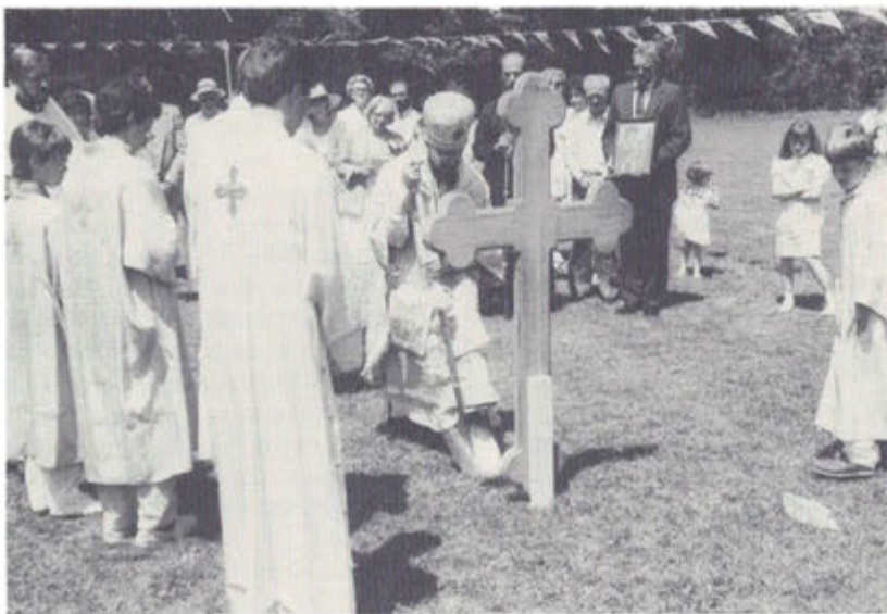
Bishop Herman breaking ground for the new Church.
